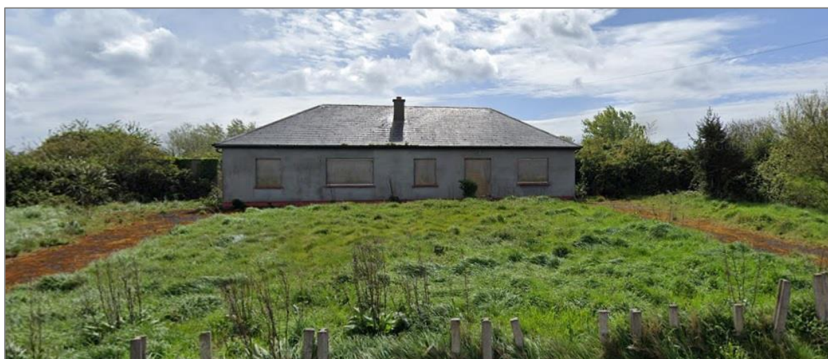
Figure 13.10 Bungalow to be demolished
